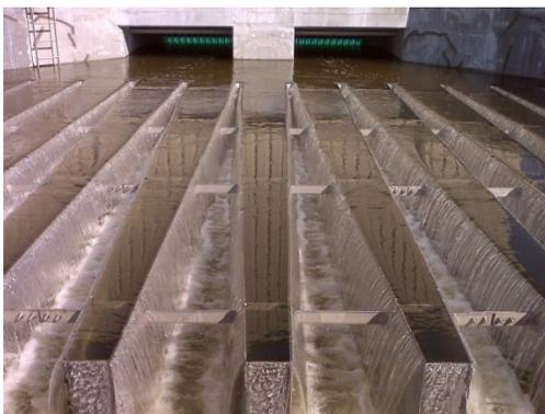
*Final Effluent – Disinfected by Ultraviolet Light*
