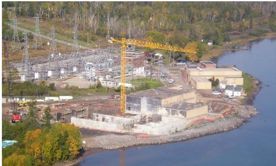
Bare Point Water Treatment Plant Expansion Project
