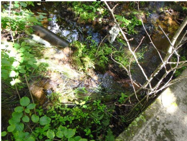
Image 13: Iron Pipe intersecting Retaining Wall facing N
