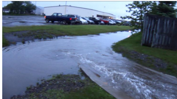
Figure 6 – Discharge from the Intercity Pumping station to the Beverly concrete lined ditch looking north east toward the Moose Hall
