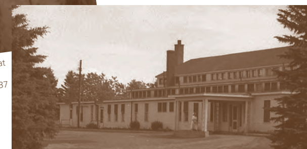
Ontario Hospital Fort William, 1937
