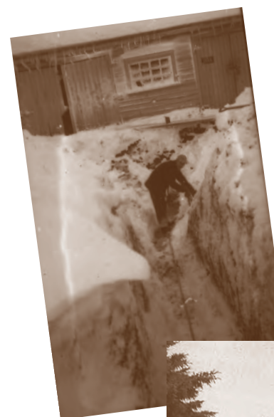
Water problems at Ontario Hospital Fort William, 1937
