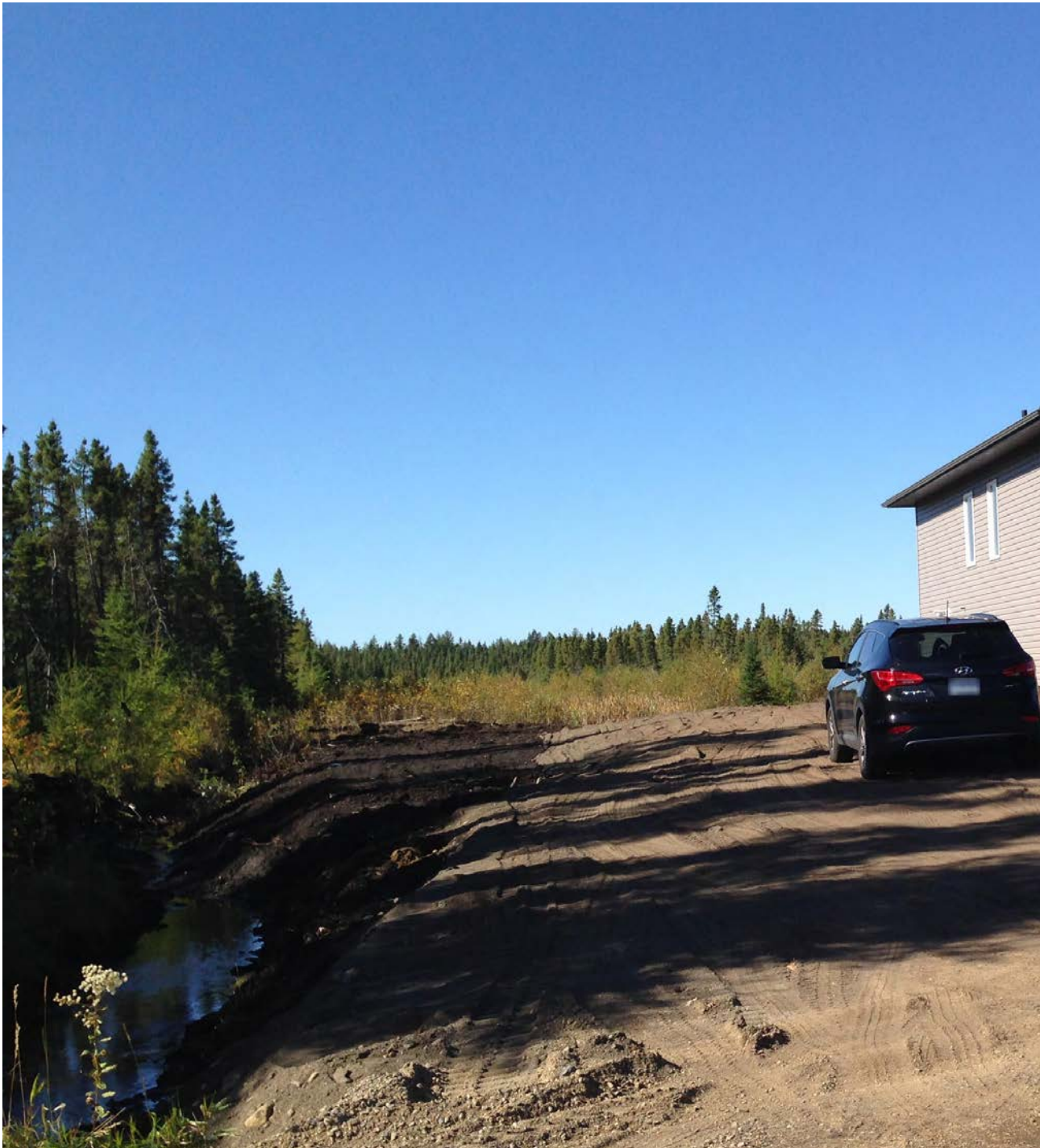
Figure 11 - Recent home construction in upper watershed of McVicar Creek. Note wetland filling and lack of erosion control
