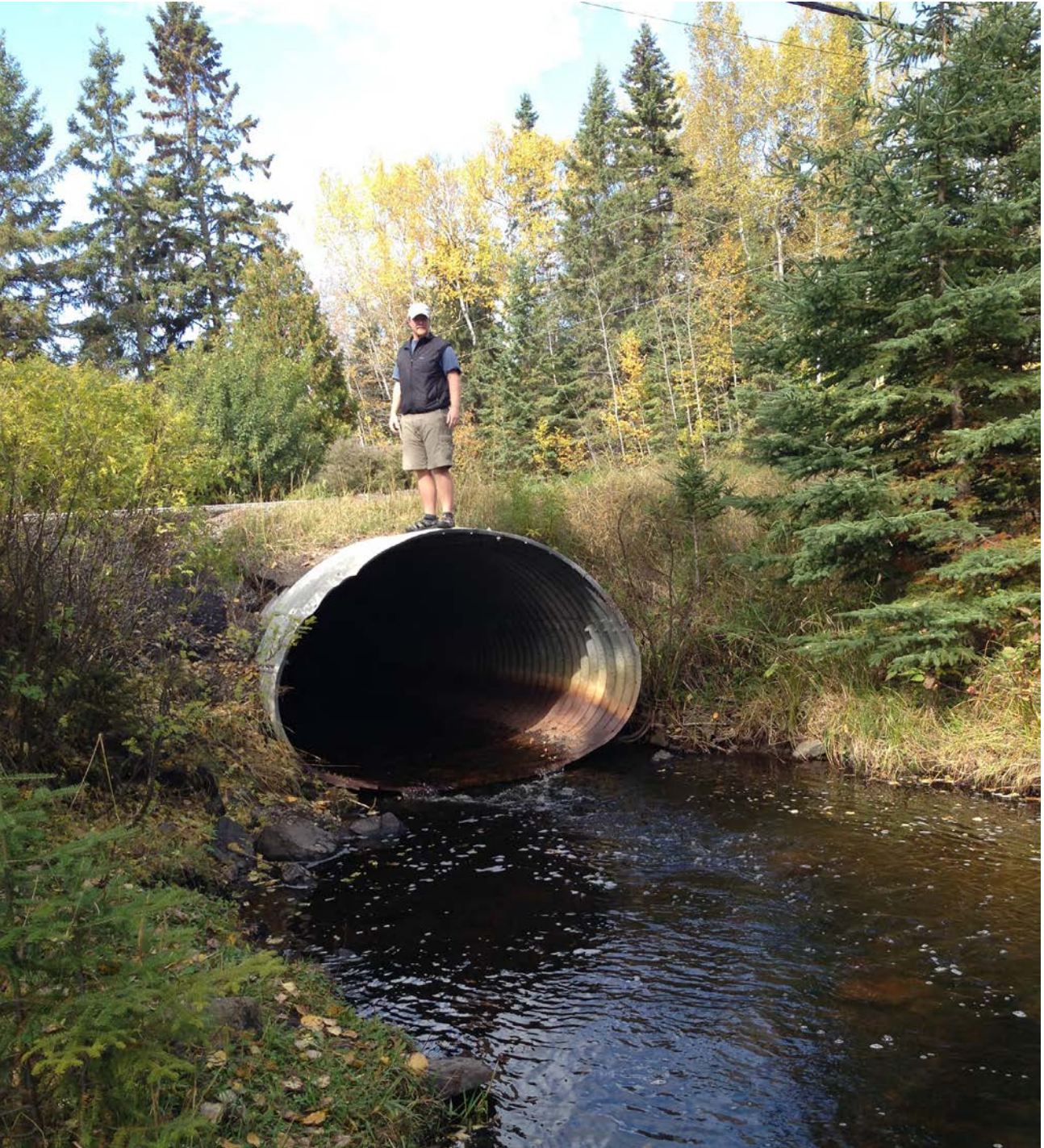
Figure 13 - Slightly perched crossing in the upper watershed that may be a barrier during periods of low flow
