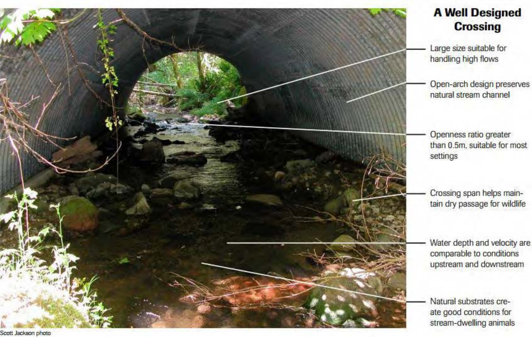
Figure 37 - Example of a well-executed crossing design. (Image courtesy of the State of Massachusetts Division of Ecological Restoration.)
