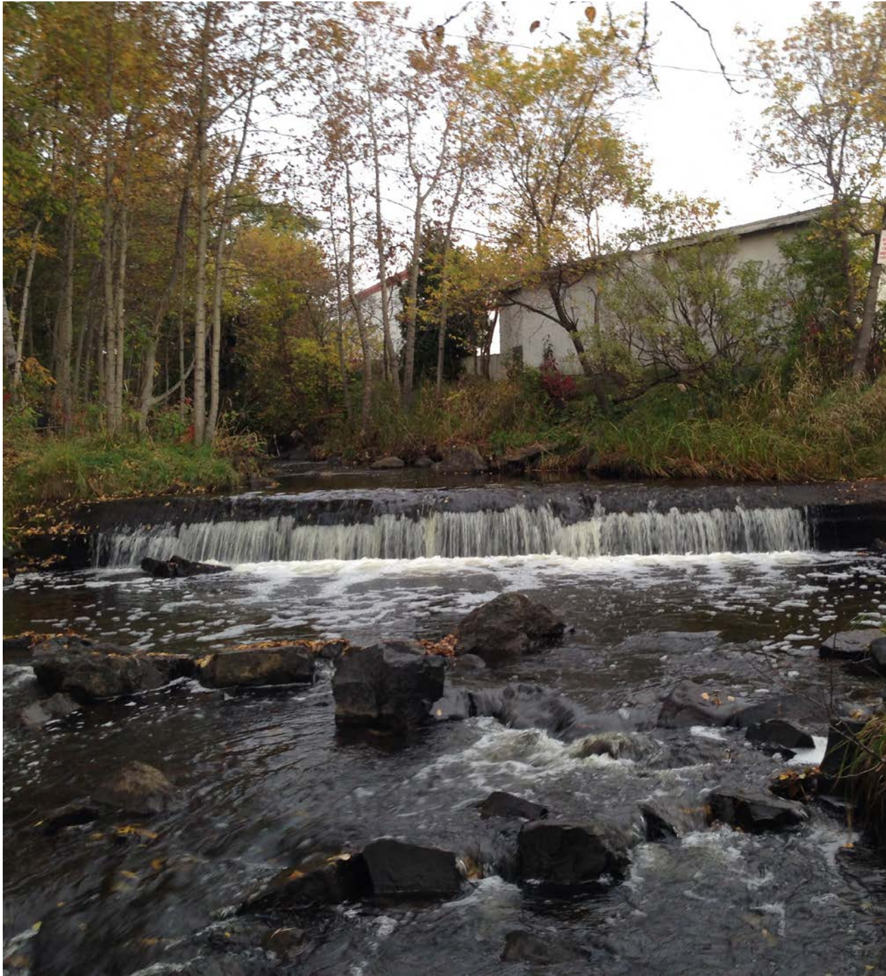
Figure 14 - Utility crossing downstream of Cumberland Street. These obstructions, which are common throughout McVicar Creek are not thought to be barriers to game fish, but may be to the invasive Sea Lamprey.
