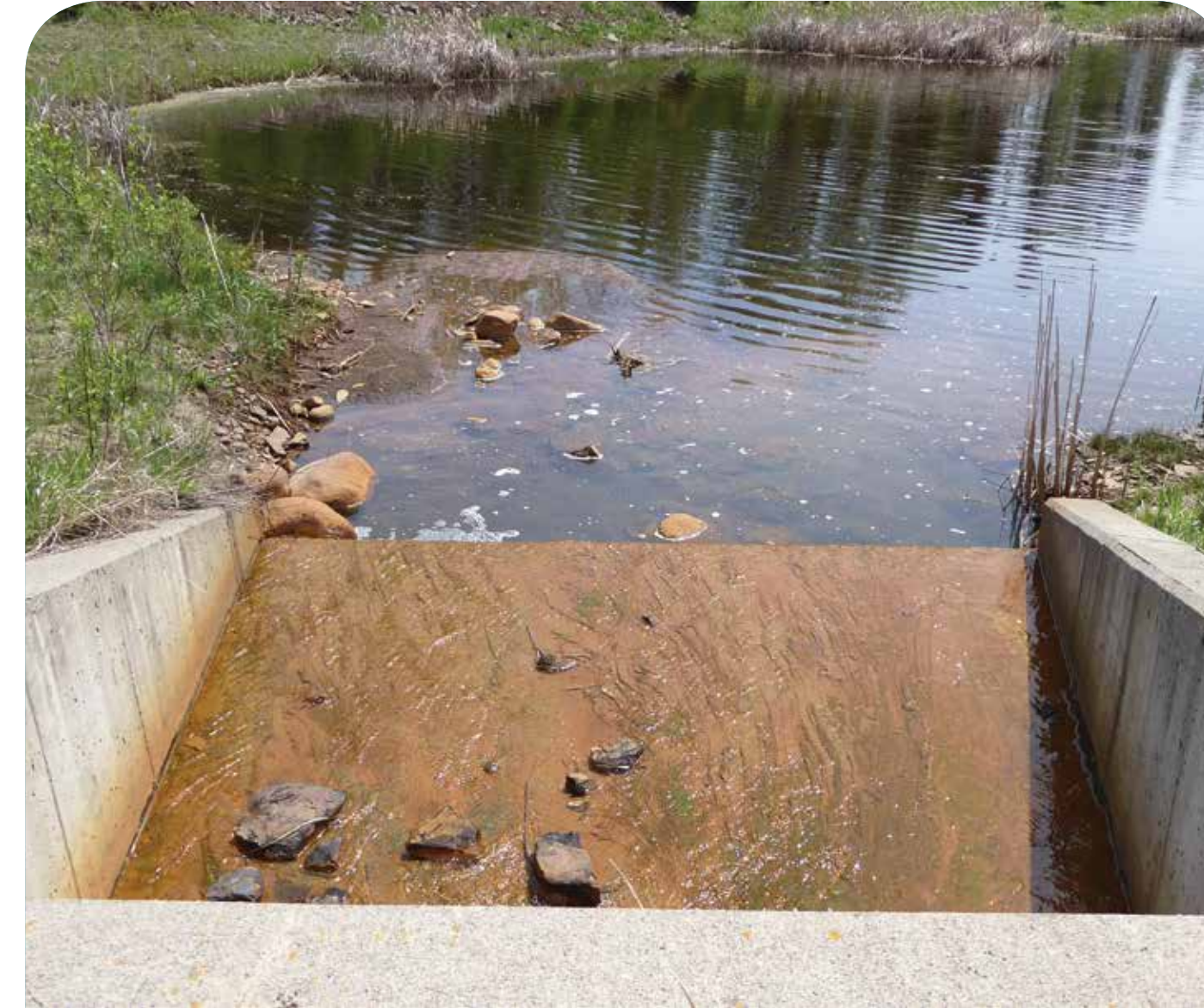
Inlets and outlets
