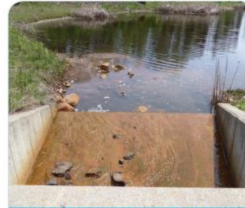
Inlets and outlets
