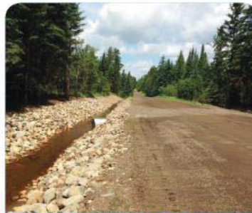
Ditches and Culverts
