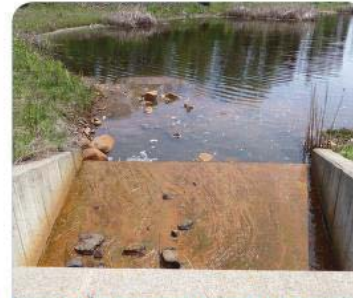
Inlets and outlets
