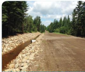
Ditches and Culverts
