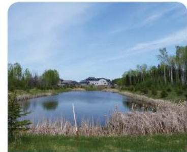
Stormwater treatment facilities, including Green Infrastructure
