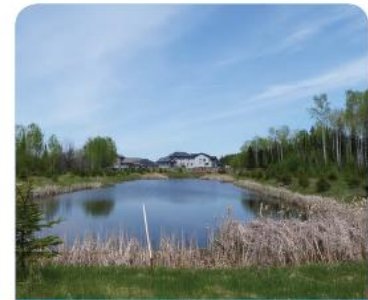
Stormwater treatment facilities, including Green Infrastructure
