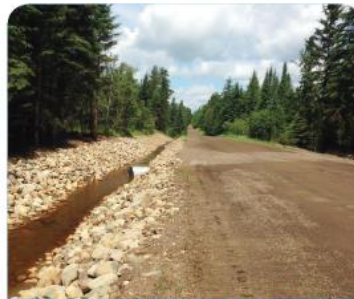
Ditches and Culverts
