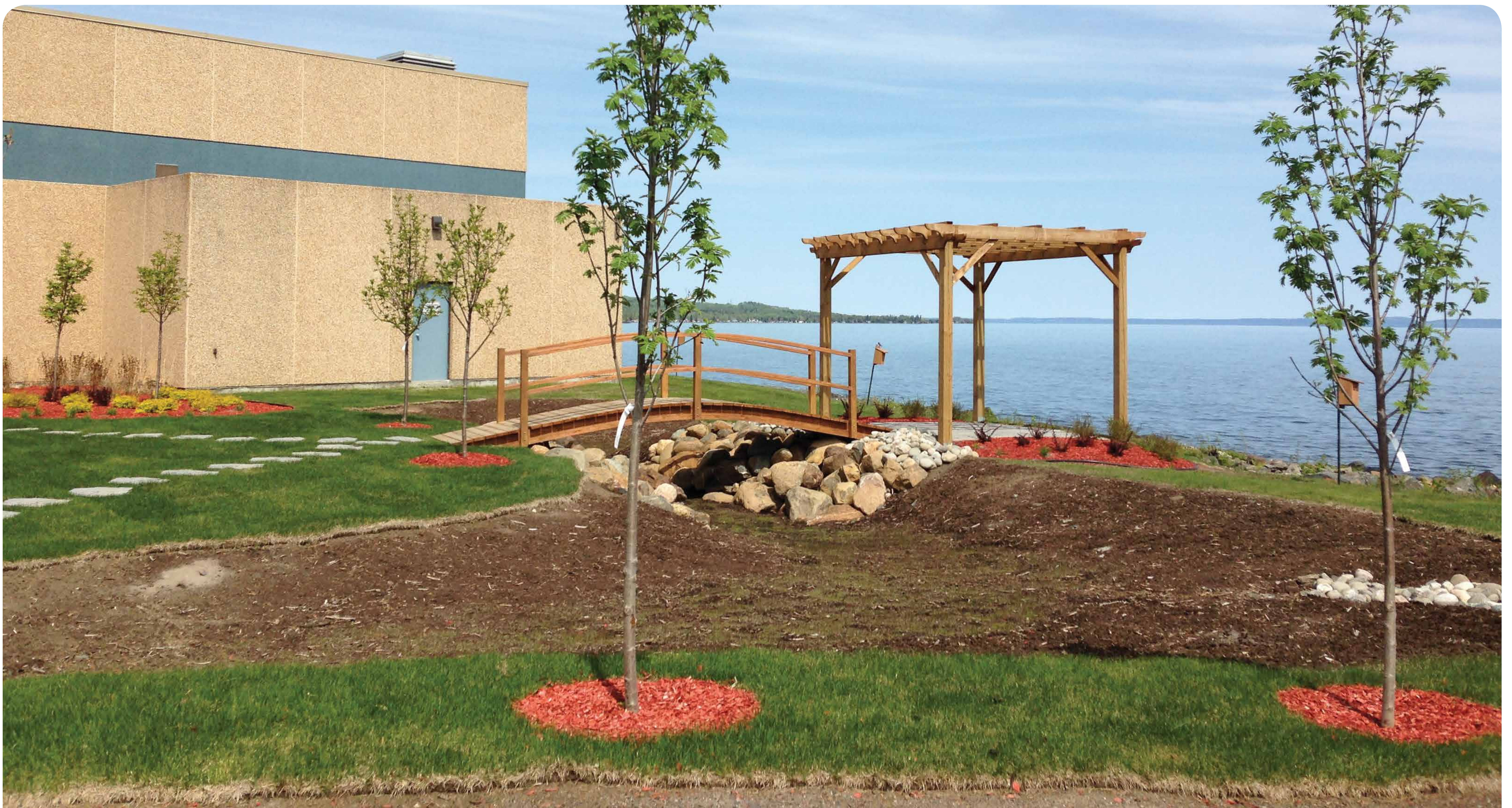
Green Infrastructure at the Bare Point WTP
