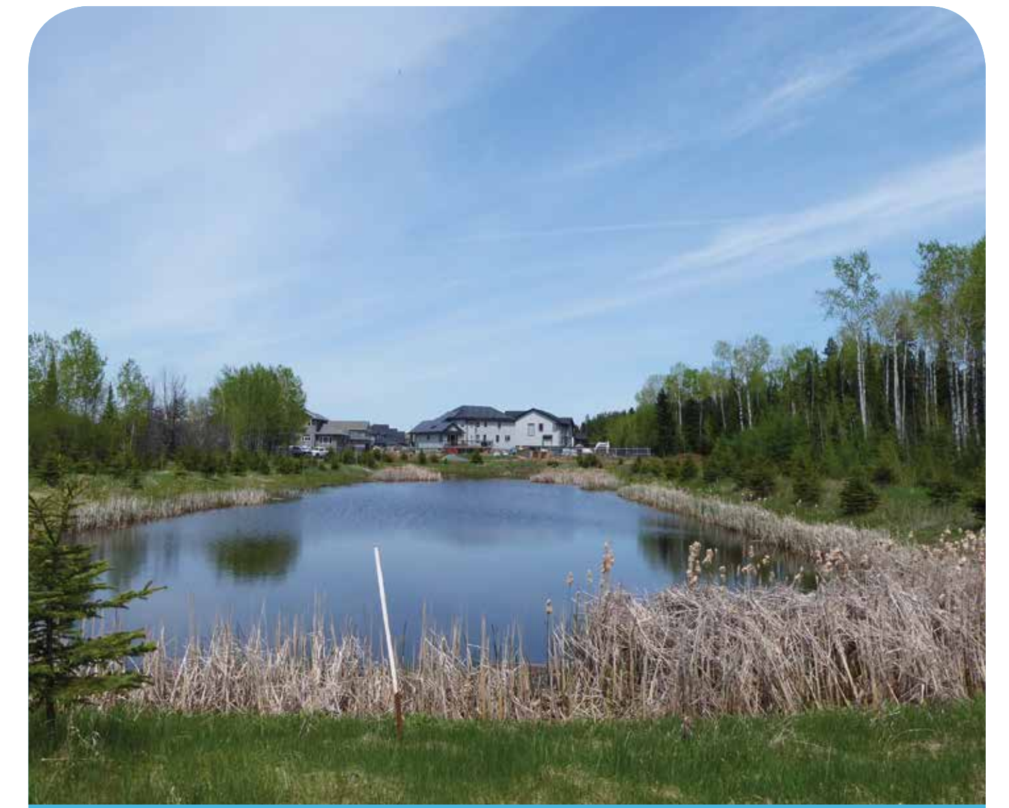
Stormwater treatment facilities, including Green Infrastructure
