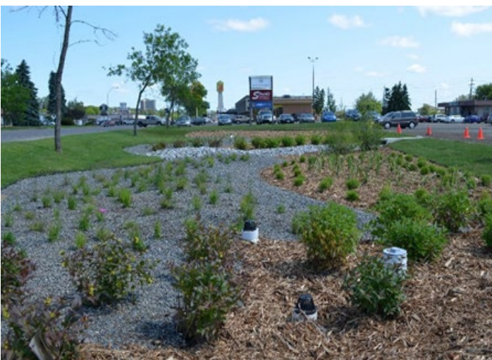
Example of Low Impact Development measures on the west side of Memorial Avenue at High Street
