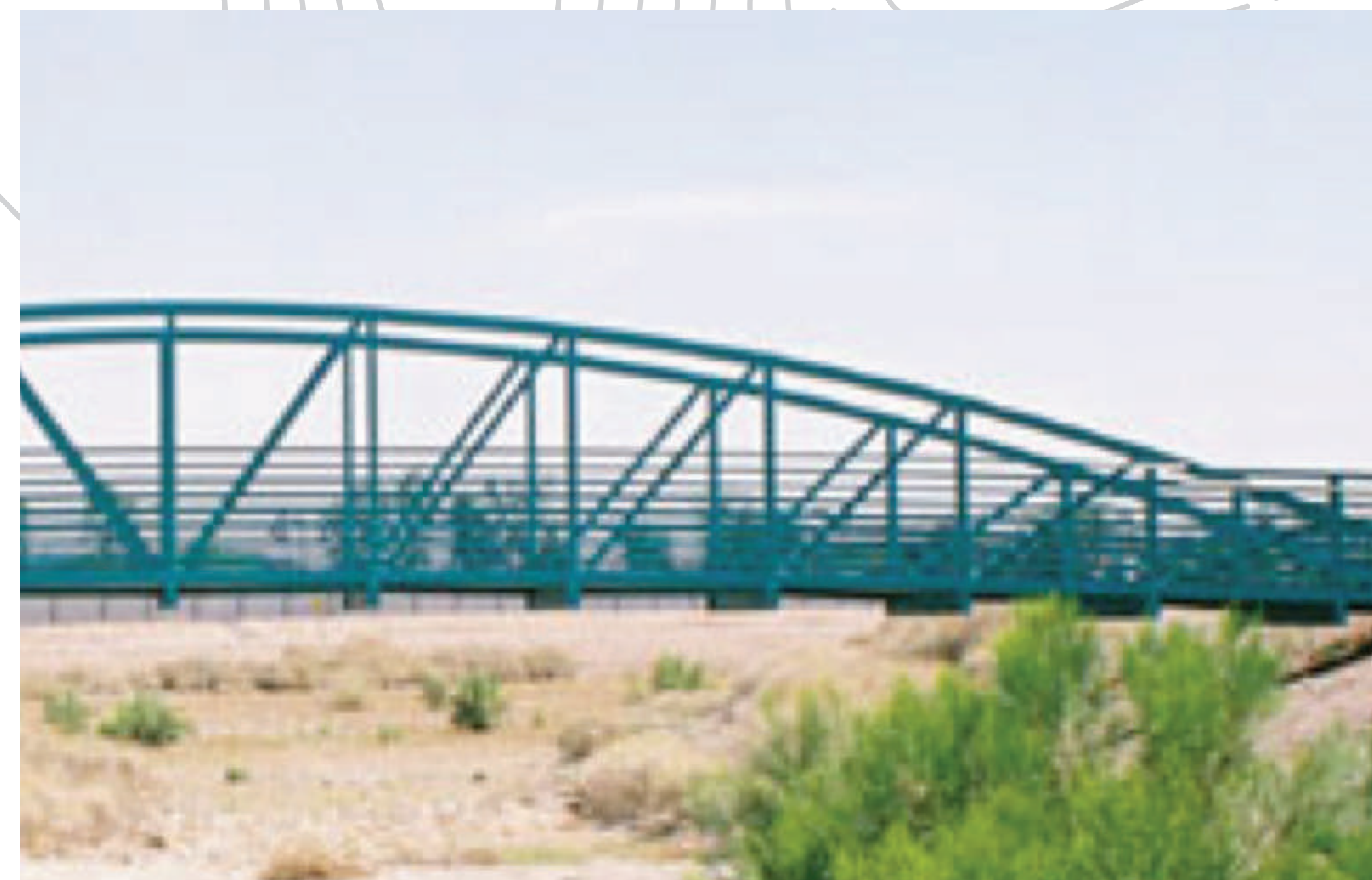
EXAMPLE OF PAINTED STEEL BOWSTRING TRUSS
