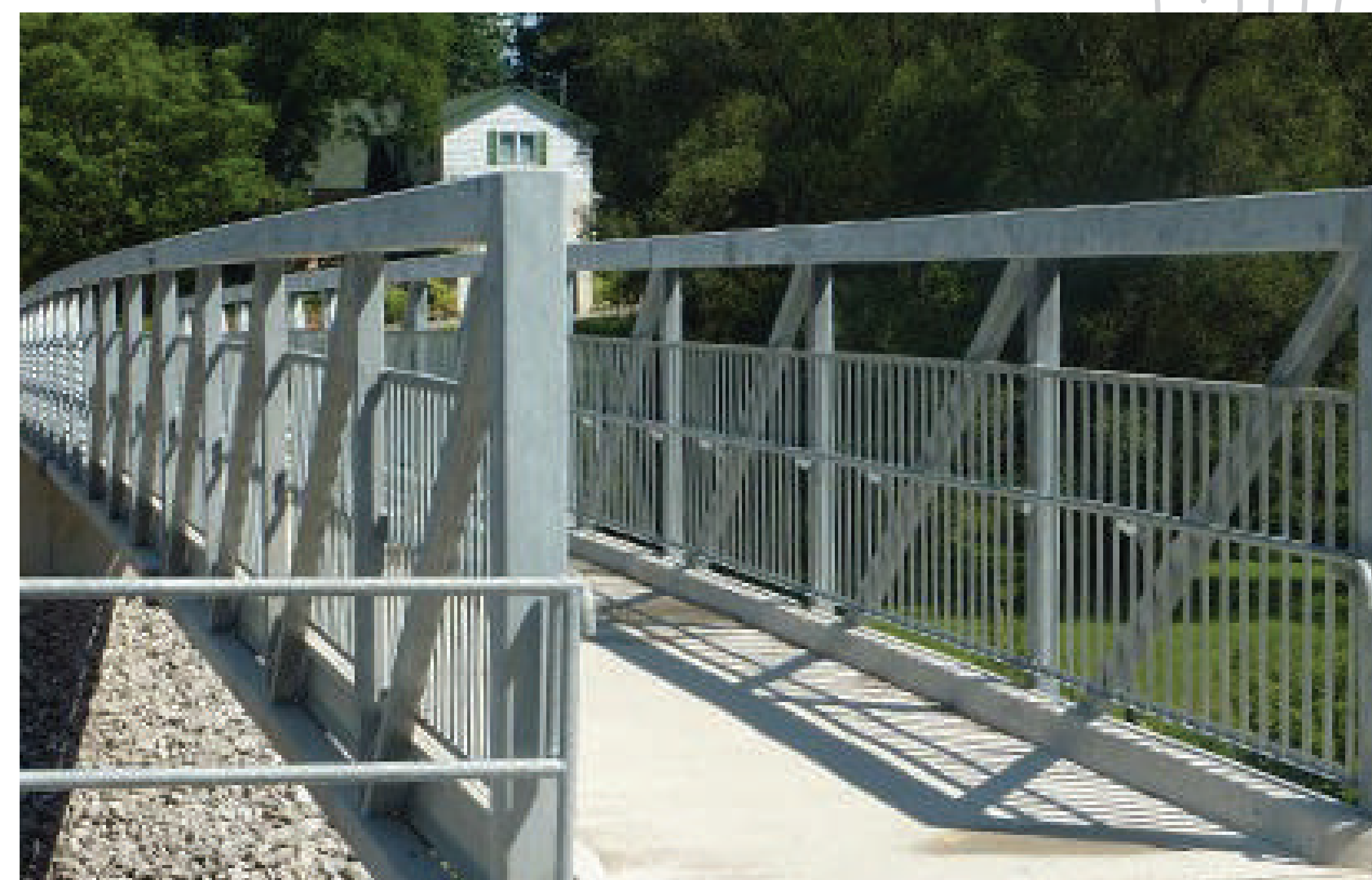
EXAMPLE OF GALVANIZED STEEL PRATT TRUSS
