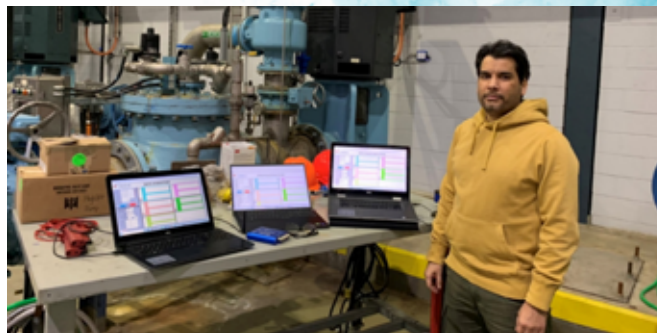
Dr. Mohamed Ahwiadi, Lakehead University Department of Mechanical and Mechatronics Engineering, stands next to data acquisition and analysis equipment, and the high lift pumps that vibration sensors were installed on.
