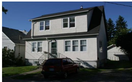
271 Harrington Ave. Built: 1940
