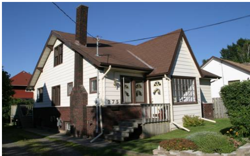
275 Harrington Ave. Built: 1929
