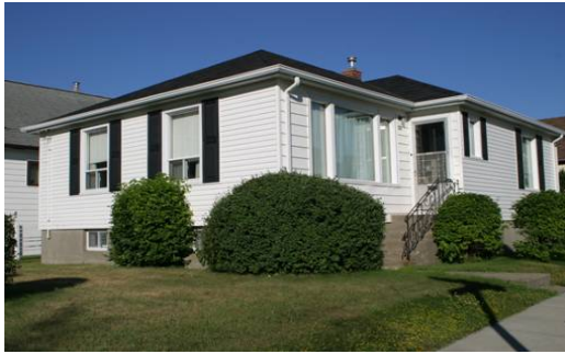
255 Harrington Ave. Built: 1950
