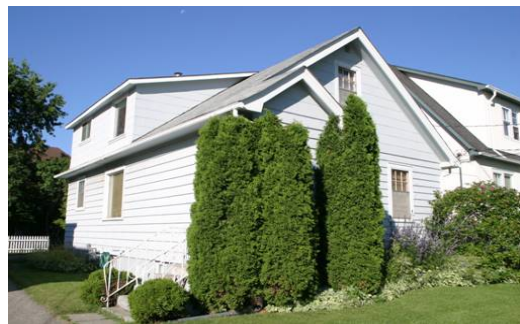
267 Harrington Ave. Built: 1936
