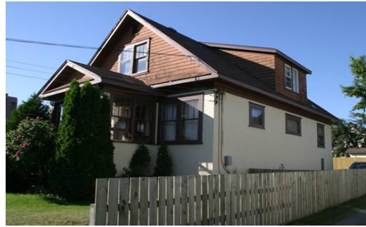
263 Harrington Ave. Built: 1936
