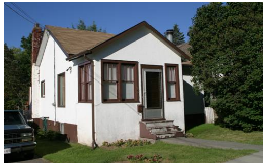
279 Harrington Ave. Built: 1924*
