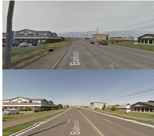
Exhibit 1.2: Balmoral Ave before and after rebuild
