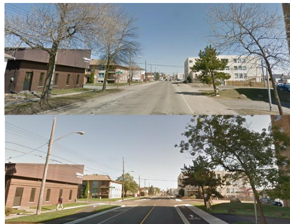
Exhibit 1.3: Court St before and after rebuild.
