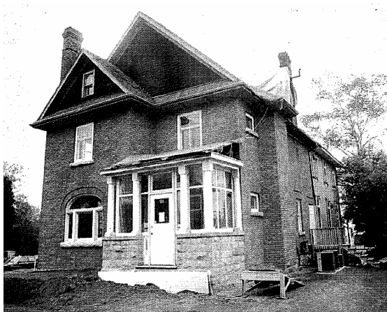
McKibbin House, during restoration 1992
